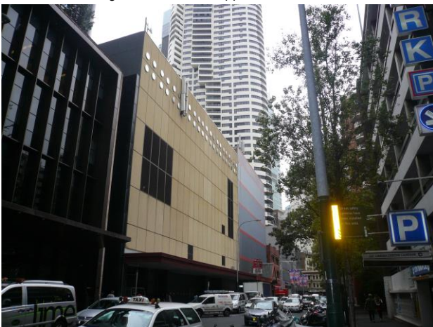
View of the site from Kent Street
