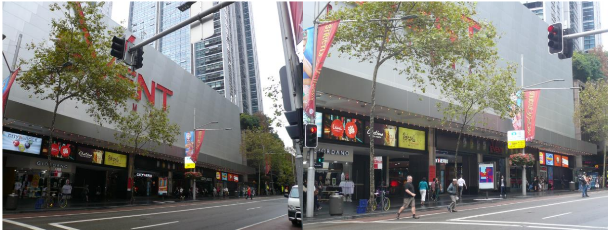
Views of the site from George Street
