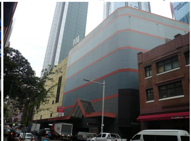
View of the rear of the Hoyts Cinema Complex on Kent Street, located adjacent to the site
